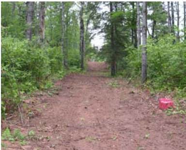
Finished work to re-route Fish Lake trail.
